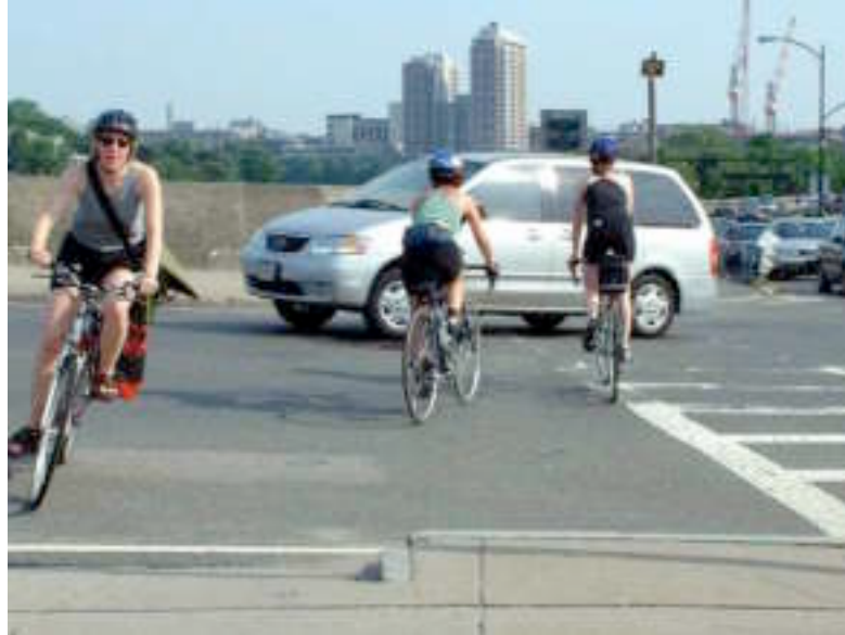
The crosswalk does not match up with the ramp, making crossing even more difficult.
